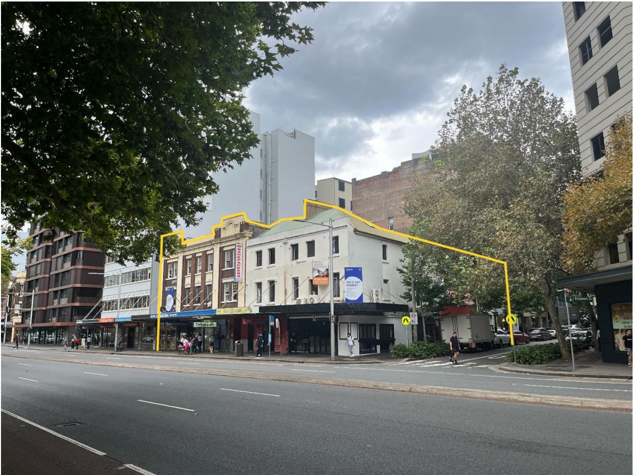
Figure 5. 232-240 Elizabeth Street, viewed from the south-west, outlined in yellow
