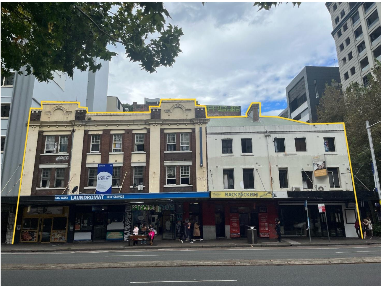
Figure 3. 232-240 Elizabeth Street, viewed from the west, outlined in yellow (Elizabeth Street frontage)
